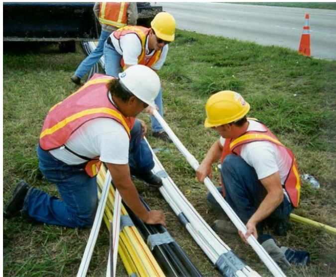
Figure 1 – Duct Installation using Mechanical Couplers
